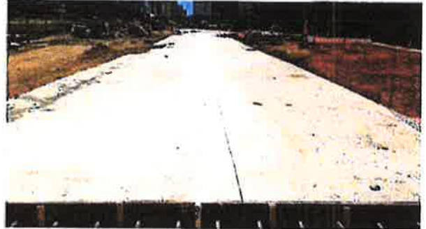
Town & Country Blvd. concrete pavement in progress—looking south
