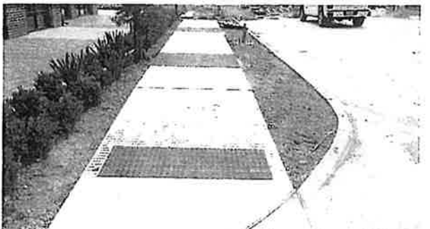
Decorative sidewalk paver inserts installed along Town & Country Way
