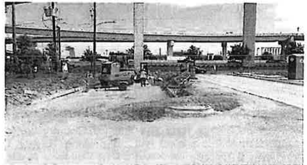
Constructing NB Town & Country Blvd. - looking north
