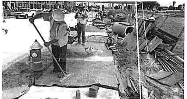
Installing decorative sidewalk paver inserts along Town & Country Blvd.
